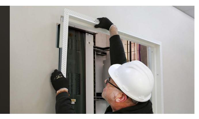
The Novista Riser Timber doorsets have been successfully fire tested in various different flexible and rigid wall constructions, and as a result, they can be installed in blockwork, timber stud or metal stud walls appropriate to the required fire certification.
