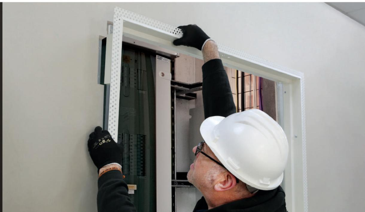
The Novista Riser Timber doorsets have been successfully fire tested in various different flexible and rigid wall constructions, and as a result, they can be installed in blockwork, timber stud or metal stud walls appropriate to the required fire certification.
